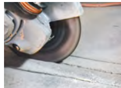
Creation of traces on reinforced concrete.
